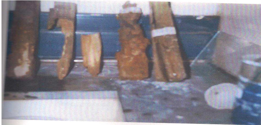
Figure 2: Woods infested by termites
